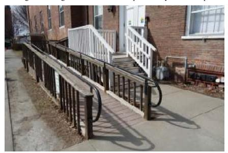
handicap ramp are otherwise in good condition. The decking on the handicap ramp is composite and does not require maintenance. The porch is budgeted for a full round of repairs in year 12.
