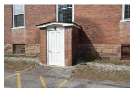
The basement entrance was added to meet egress codes from the basement. It has had problems with water entering the structure and draining into the basement. This is partly due to the drainage around the building and to the location of the entrance directly under the drip line of the large main
