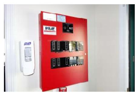
34 Elmwood Ave. – This building has had some rewiring as recently as 2003. The panel is in good condition. There were no visible wiring defects or problems reported. The wiring and lighting is budgeted for a round of upgrades in year 6.
