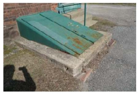
The storm door is budgeted for replacement in year 9. The Bilco door has extensive rust and has begun to deteriorate. It should be scraped and painted with rust resistant paint in year 1. Its life is limited due to the rust and replacement is budgeted in year 9.
