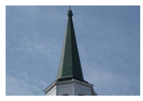
Southgate also recommends a review and repairs to the lightning protection. The most recent upgrades were in 1999 and it seems reasonable to confirm that it is still working properly. This is an unusual skill and should be performed by a specialist.
