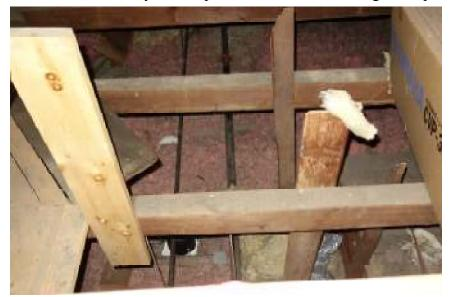
Meetinghouse – This building has several different attics and wall profiles. The original building has an insulated attic over the main ceiling. It contains a mixture of fiberglass and vermiculite. There is a concern that the vermiculite may
