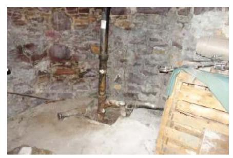
30 Elmwood Ave. – This building has sewer and drain lines that date from before the 1994 renovations. There are extensive hubbed iron drain lines that are over 50 years old (probably over 75 years old) and are prone to failure. These problems may extend beyond the building to the
